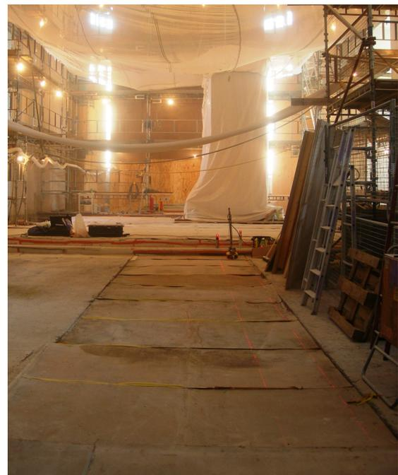
Figure 5: Relatively good laser beam visibility in daylight with additional artificial lighting
