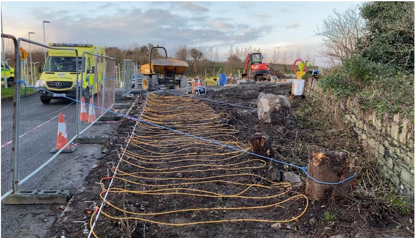
Figure 3: ERI survey across Area 1 – a 18 m x 6 m strip of land. Hospital ambulance bay to the left; construction of new helipad in background; an extant portion of the 1847 Cholera Field Wall on right.
