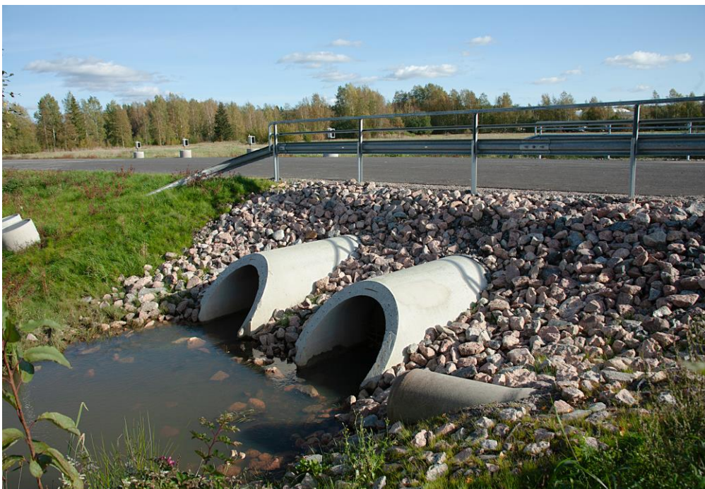
Figure 1: The large pipes below the bridge. The measurement line ran along the bridge.
